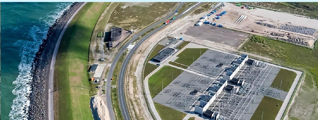
Offshore wind landfall
